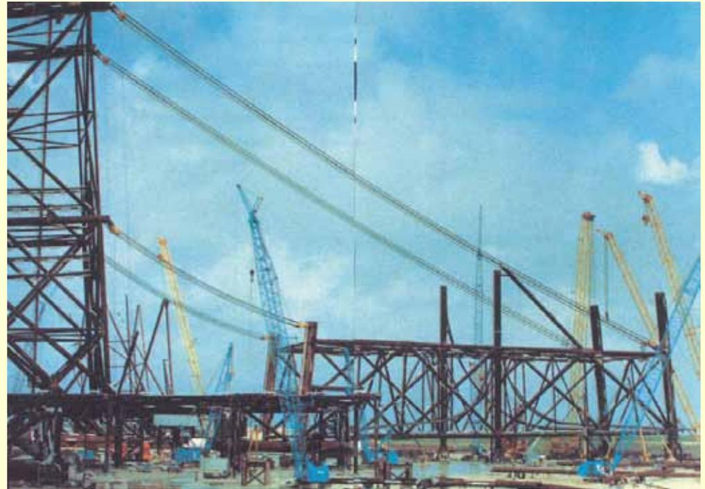
**Bullwinkle “**core-block**” method due to larger dimensions of base structure. At required height, crawler cranes provide inadequate lift capacity**
