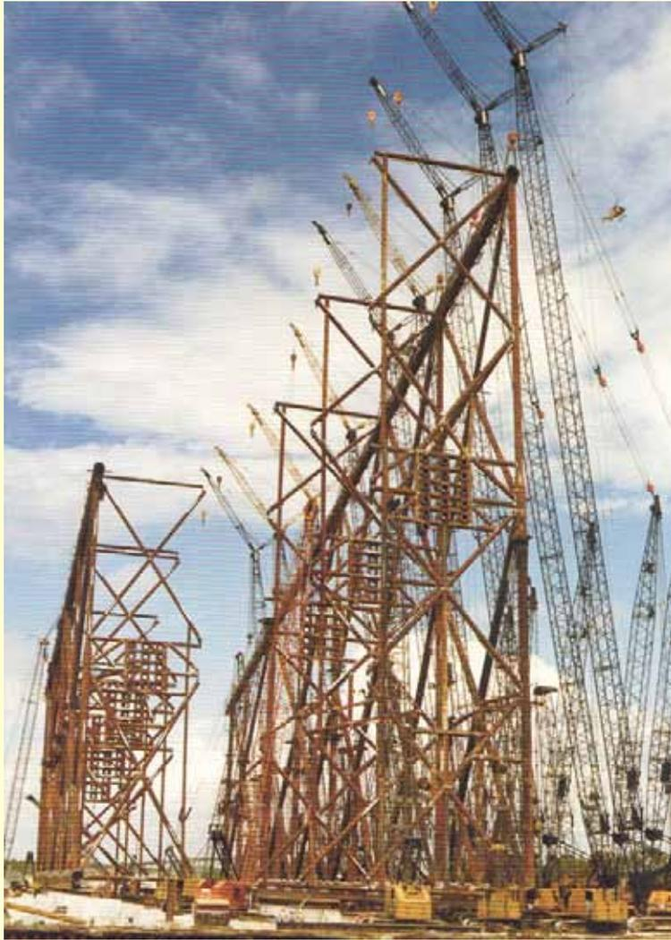
**Reach and capacity of crawler cranes sufficient for roll-up of bent**
