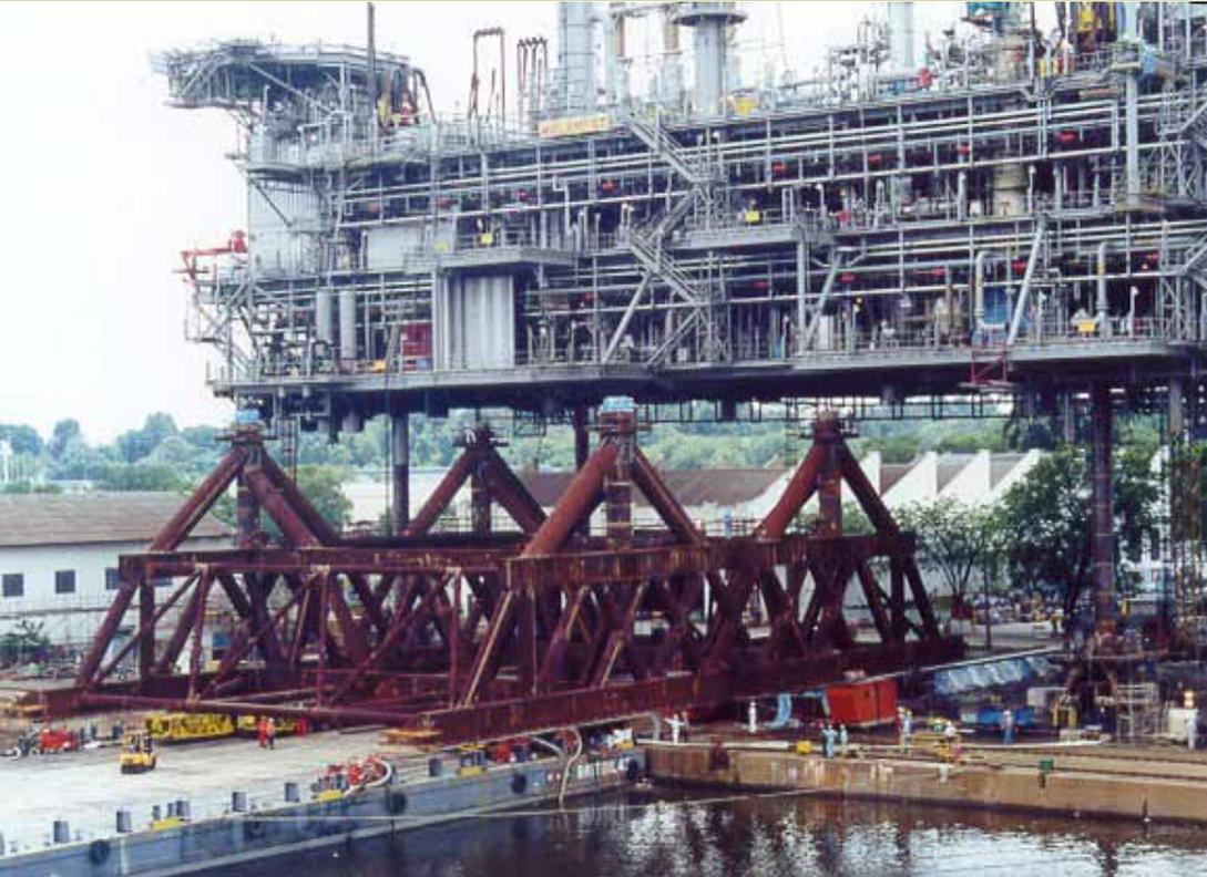
**Positioning transport truss below jacked-up integrated deck**
