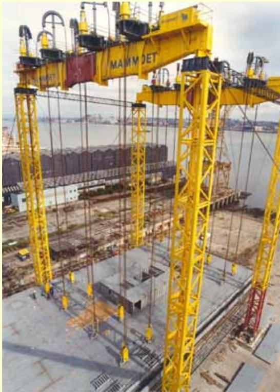
Lifting using synchronised strand jacks
