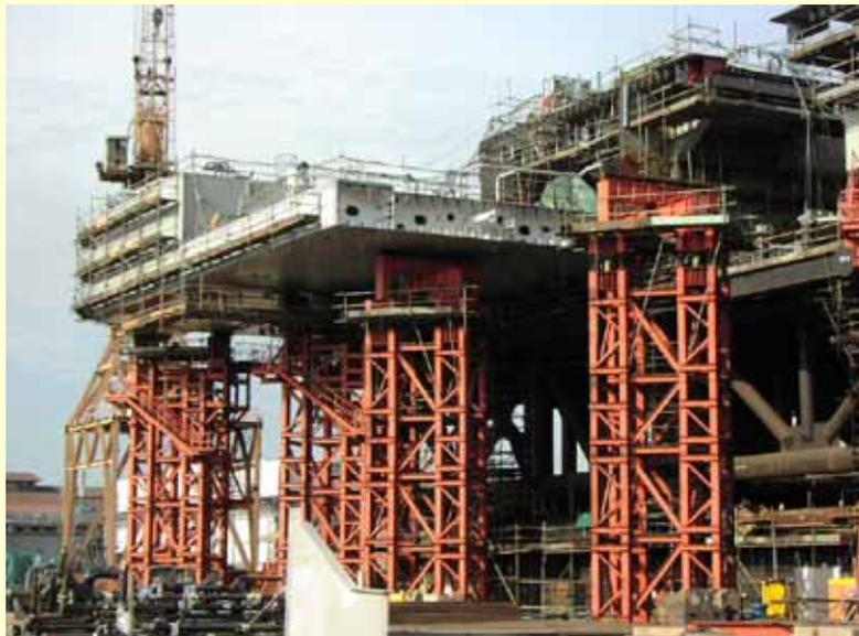
**Lifting of module ; support towers; and support truss for integration of deck modules**
