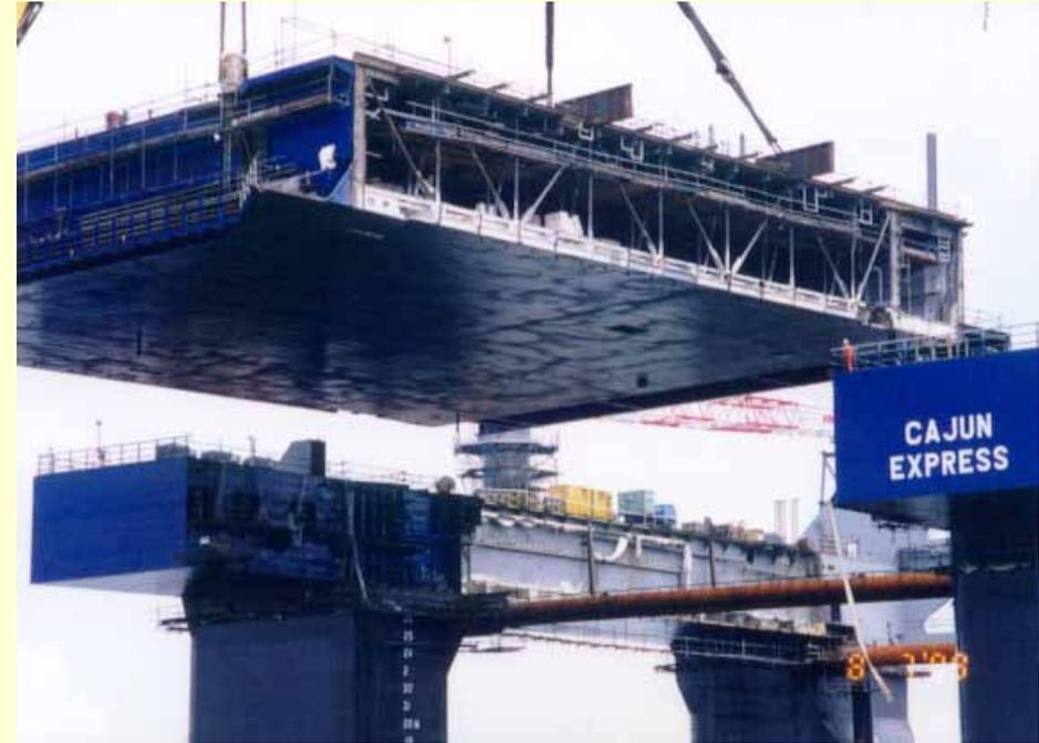
Zoomed-in view (note the temporary truss on side of block, and lift point)
