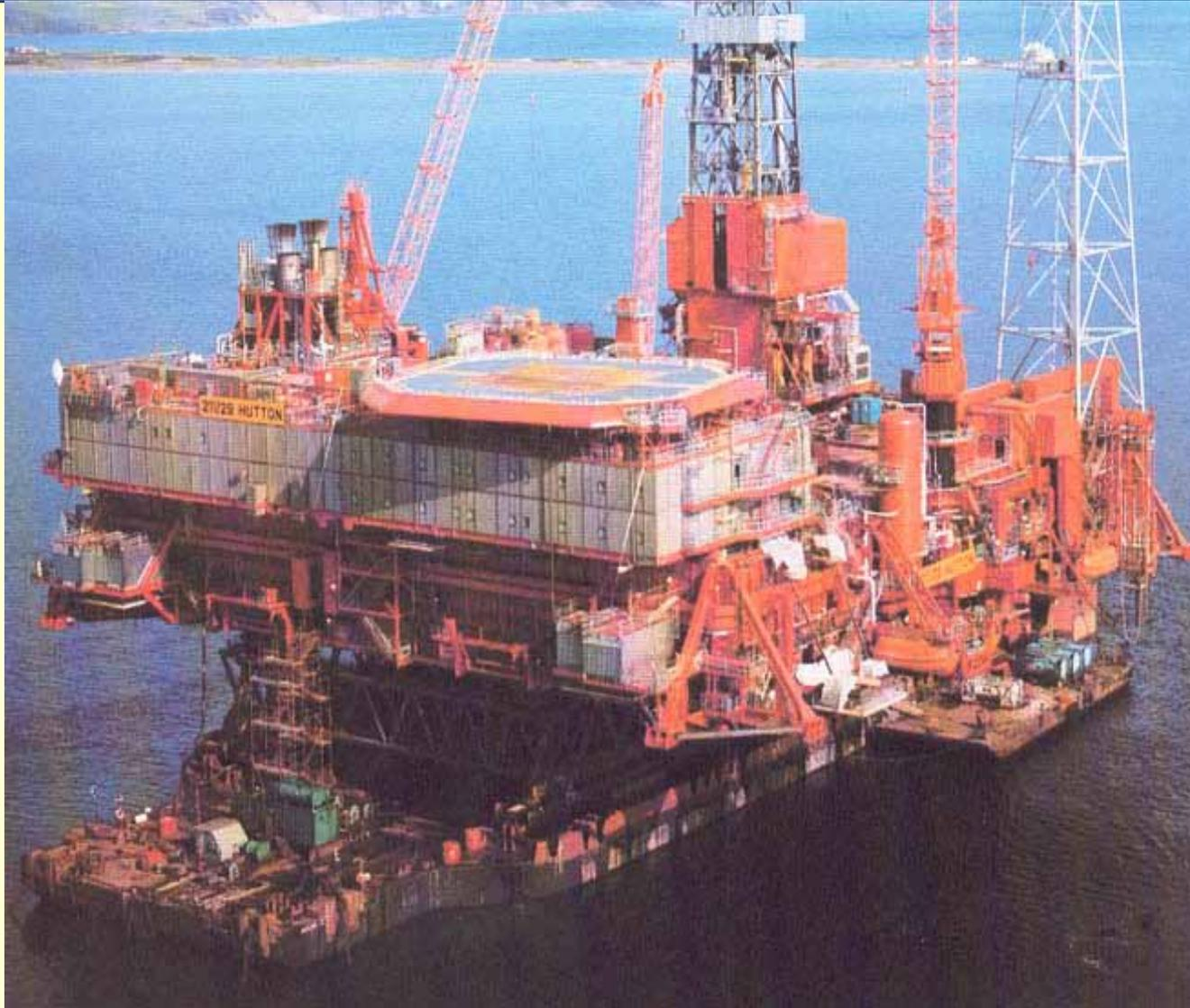
Note complex transfer truss supporting deck and large overhang on both sides of barge
