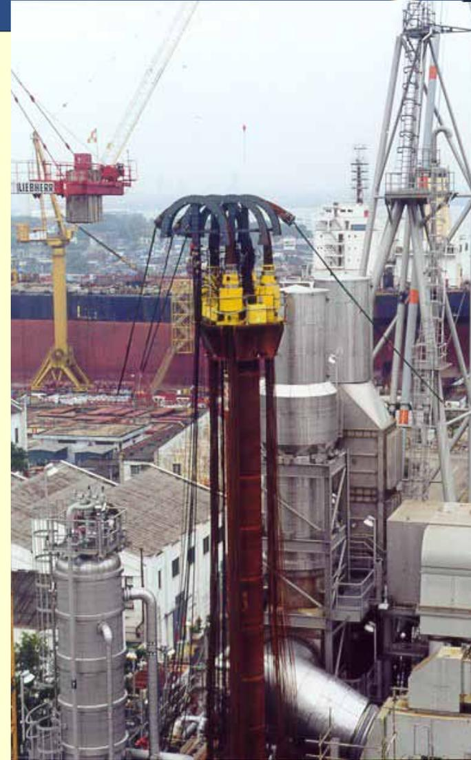
Views of vertical columns and strand jacks prior to lifting
