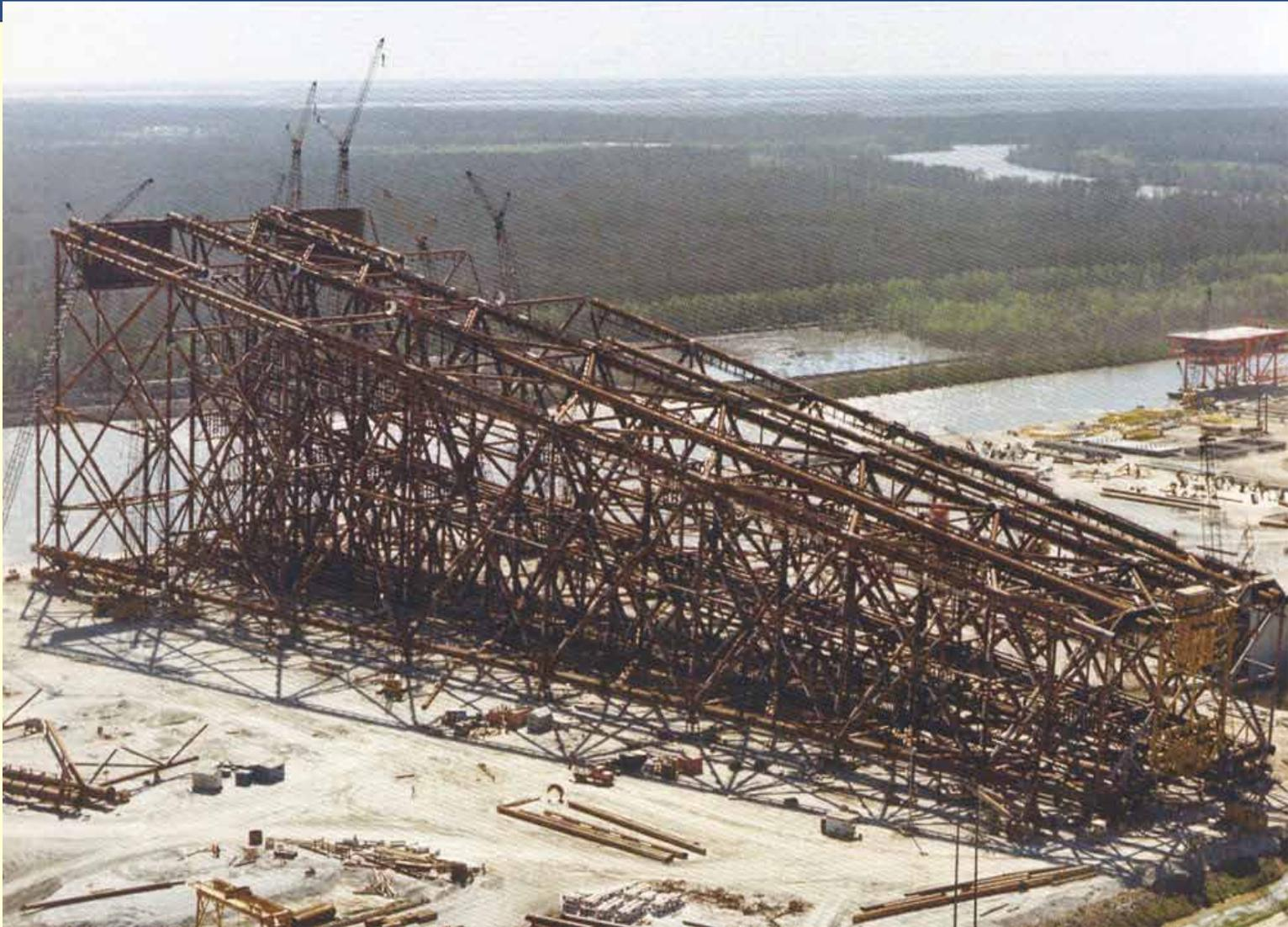
Height (to top of rigs): 327m; Weight (at launch): 26,000 tonne
