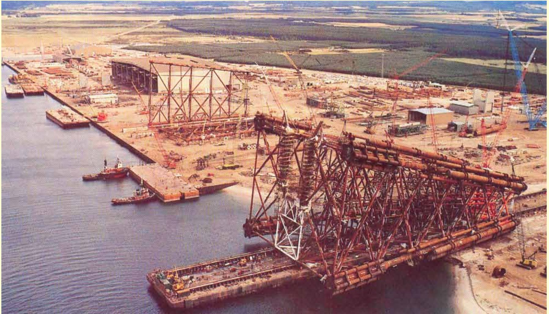
Jacket load-out (in the fore-ground), cranes and flat-top barges
