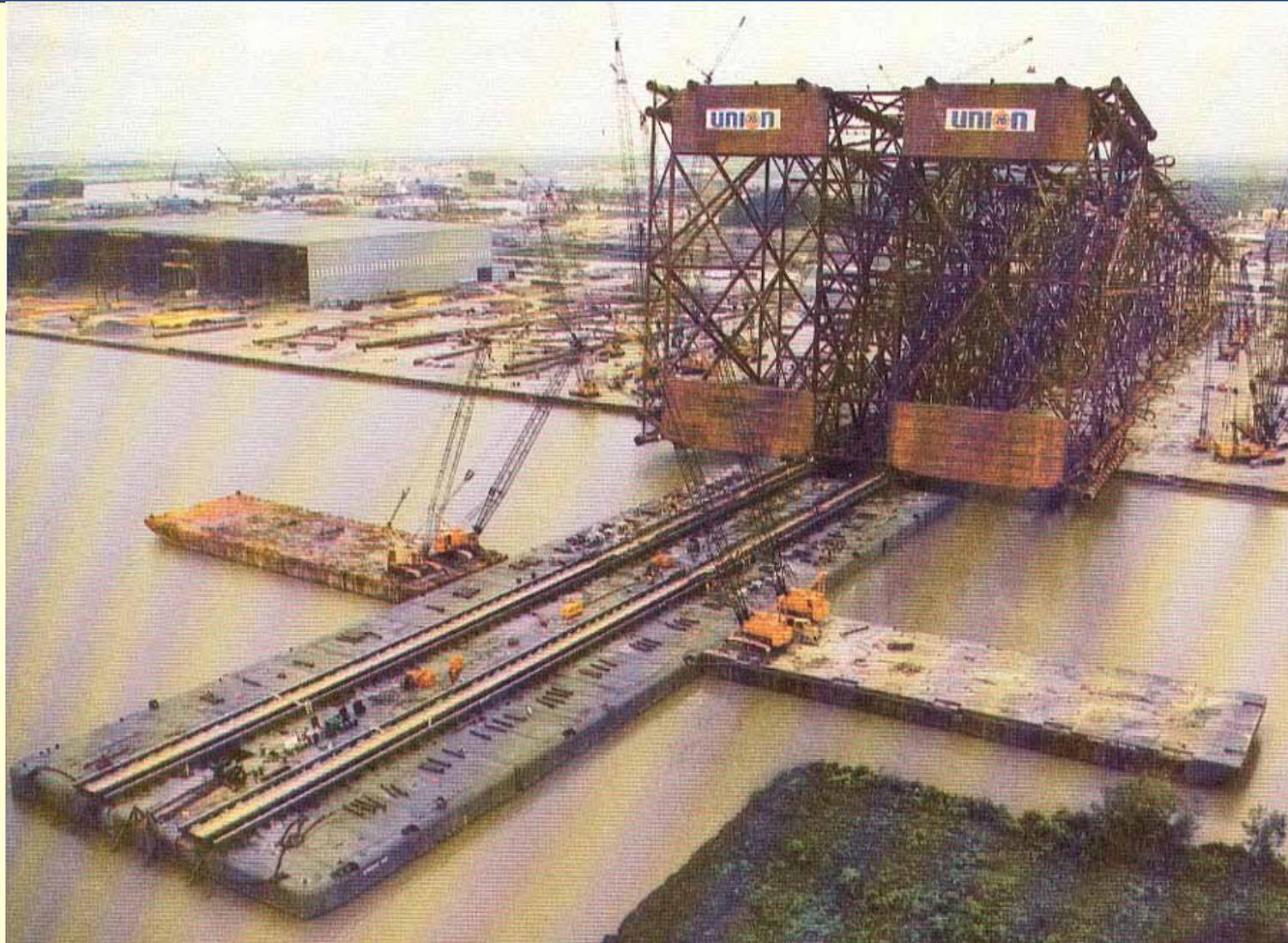
Note the 2 skid beams on barge, used for loadout and launch operations
