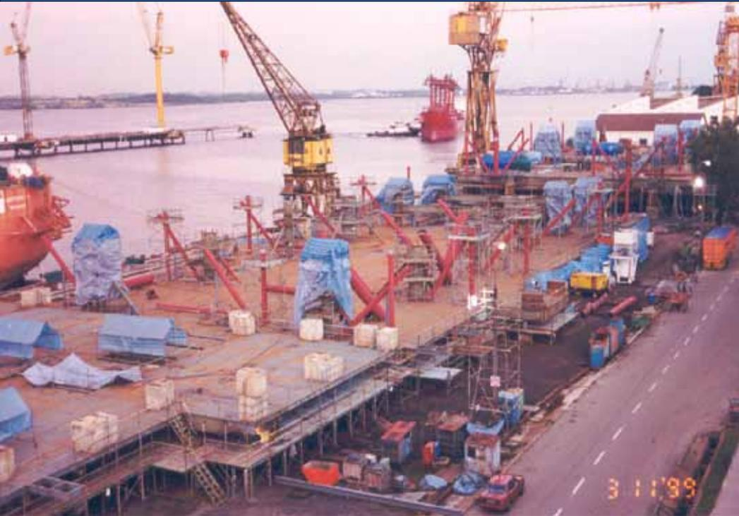
**Concurrent fabrication of three deck levels: cellar, main and weather decks**
