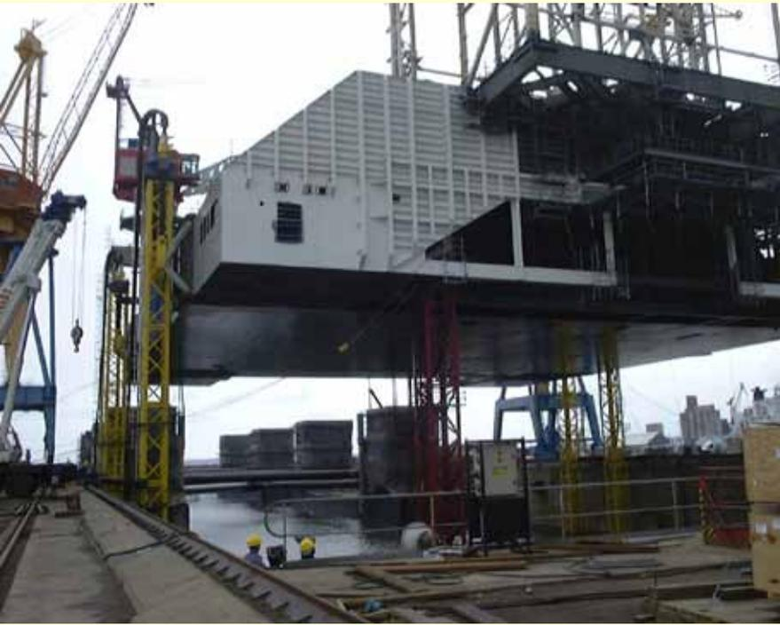
**Elevating deck structure using towers and strand jacks**
