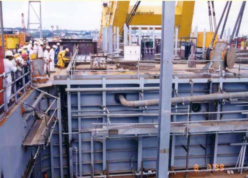
Final adjustment for fitting up; note fabricated trunnion in the fore-ground
