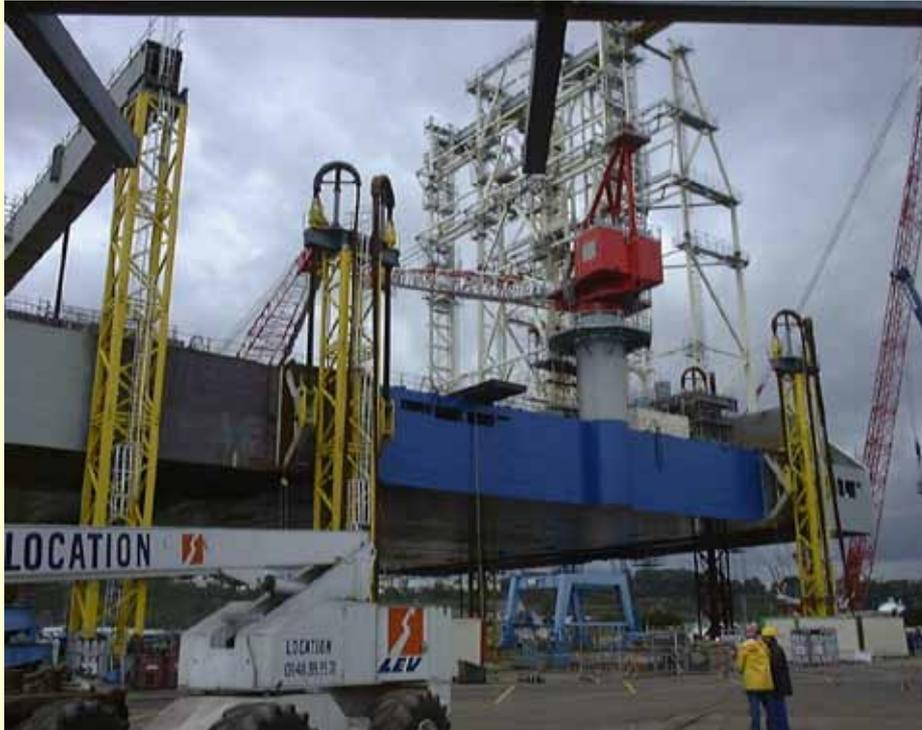
Elevating deck structure using towers and strand jacks
