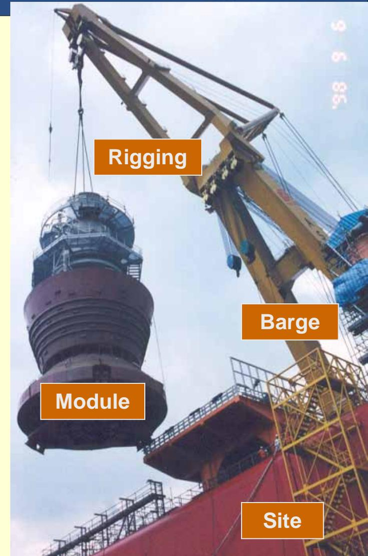
**2 stages** of lifting lower turret – off quayside & clearing side of Northern Endeavour (Laminaria FPSO)
